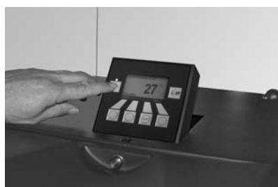
Fig. 2 Switching off FireWIN
