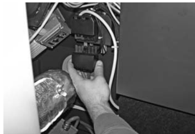
Fig. 153 Disconnecting the blower plug
