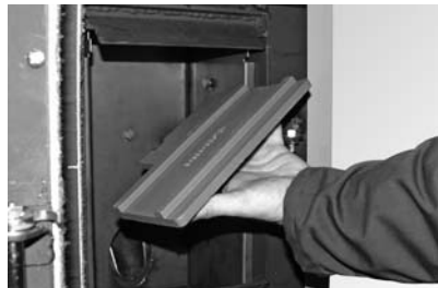
Fig. 126 Removing and cleaning the baffle plate
