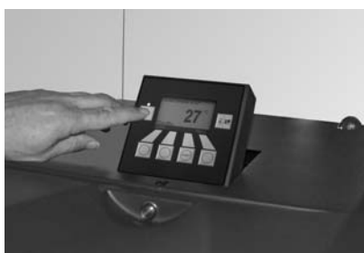
Fig. 131 Switching off FireWIN
