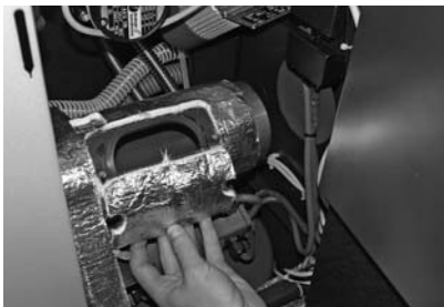
Fig. 152 Removing the wing nuts and cleaning the exhaust opening – cleaning the exhaust pipe
